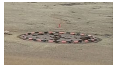
Lighted Wind Cone and Segmented Circle
